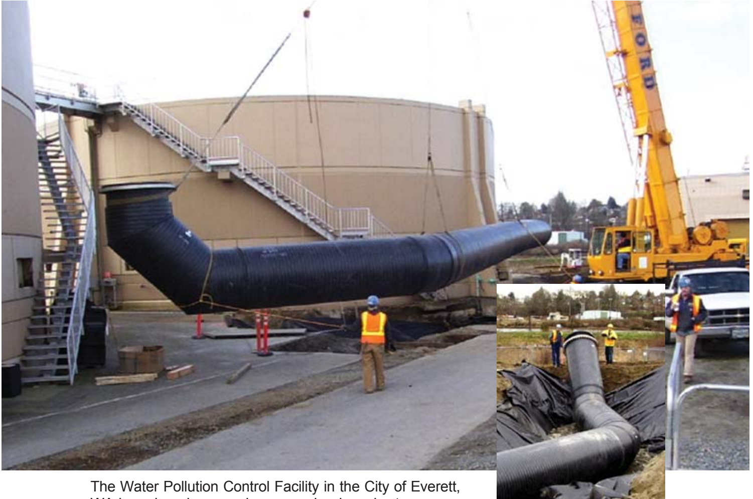
Weholite Bio-Filter installation
